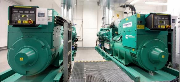
Interxion relies on state of the art saftey-engineering, e.g. extinguishing gas systems (picture above) and redundant backup generators for interruption-free continuous operations (picture below). The Frankfurt campus offers direct connections to over 450 carriers and internet service providers (small picture). Picture on the left: State-of-the-art Interxion campus in Frankfurt.
